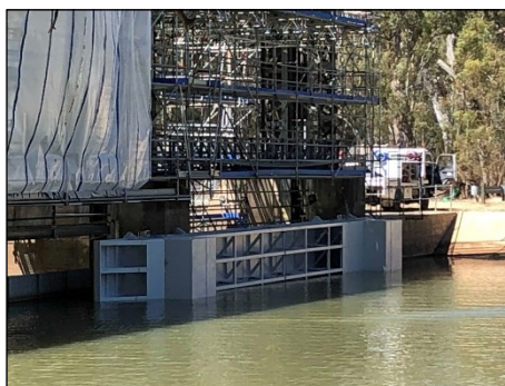
Baulk Head at Stevens Weir
